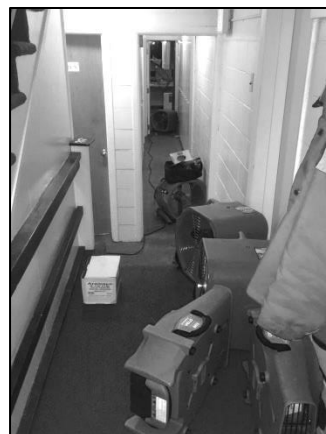
Serve Pro fans drying out the back hall way and bedrooms
