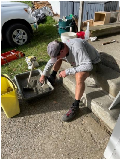
Jeff Wilks repairing deteriorated steps
