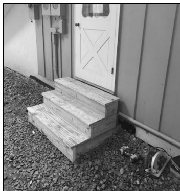
New stairs (outside kitchen door) were needed after the old ones were torn up.
