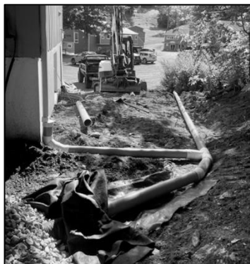
Perimeter drains for down spouts
