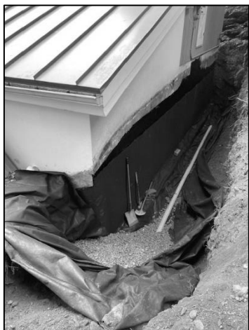
Rear footing drain
